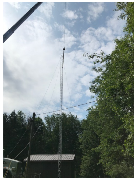
Lowering the bottom section
